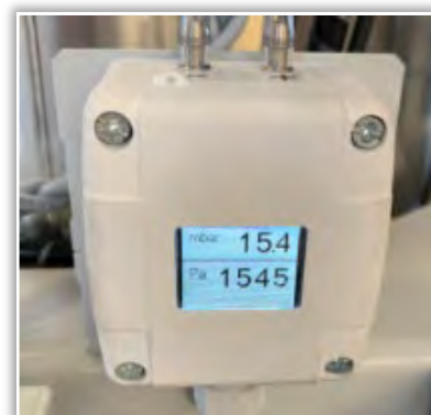
Filter state monitoring (DDMU)
